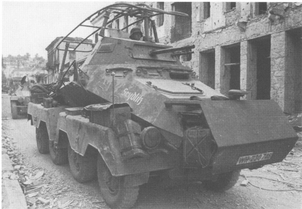
This and facing page 5th Panzer Division armoured cars in Greece: an SdKfz 232 ('Seydlitz') ( above ), 233 ('Panther') ( below ) and 221 ('Houx') ( right ) (163/327/24, 175/1265/14 and 164/369/29a).
